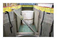
Midwest Tank Co. built this tank for the Monticello, Mn nuclear power plant to store parts that were radioactive while they were shut down for maintenace. The dimensions of the vessel are 216" dia. by 236" tall. It was built in two sections to accommodate the installation. The quick delivery of this project was essential.
